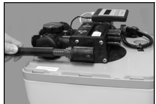
Figure 7: Connect Drain Line
