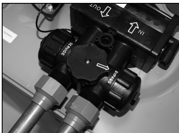
Figure 12: Bypass Valve
